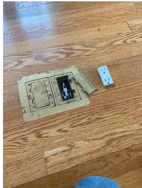
Broken Floor Outlet
