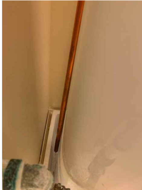
Hot Water Heater TPR Valve Discharge
